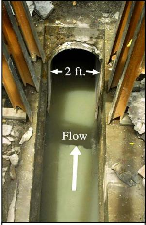
**Photo 1** – Bottom of access pit, showing end of liner in narrow duct, direction of sewage flow, and steel legs of overhead tower.
