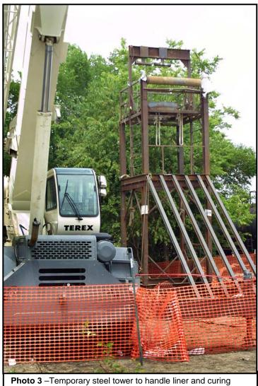
**Photo 3** –Temporary steel tower to handle liner and curing materials for the cured-in-place sewer duct relining project. The crane was used to lift fallen workers from the pit.
